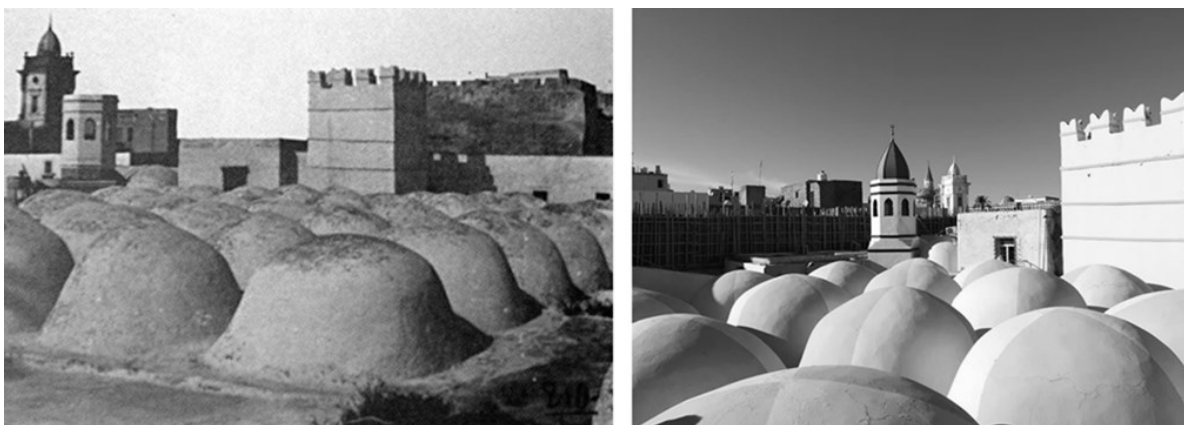
Figure 11. Left—the Al Nakah mosque's original roof domes. Source: Shaglouf, et al. (1980, p. 41). Right—the applied changes to the mosque's roof domes. Source: OCTAB's Facebook page (Accessed October 17, 2020).
