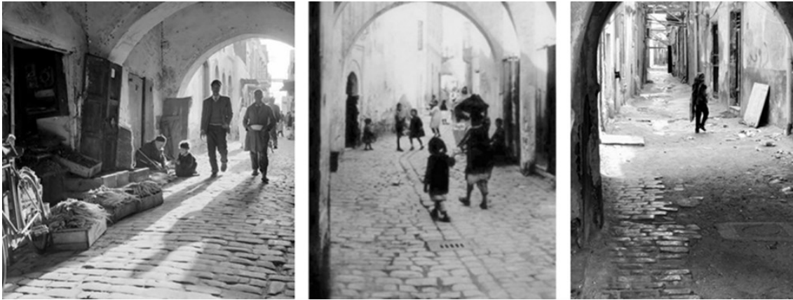
Figure 13. Left—long-lasting pavement style of Tripoli's old city streets with an interlocked straight pattern. Middle—informed approach using a narrow line for installing sewage and water systems, minimizing damage to the existing pavement. Right—uninformed approach caused significant damage to large sections of the original pavement. Source: Courtesy of Mr. Nasser Gurgi.
