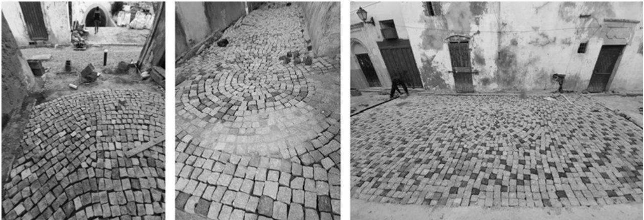
Figure 17. The imposed circular pavement pattern style using cobblestone and the arbitrary distribution of stone units over the old city's streets and alleys. Source: OCTAB Facebook page (Accessed February 1, 2020).
