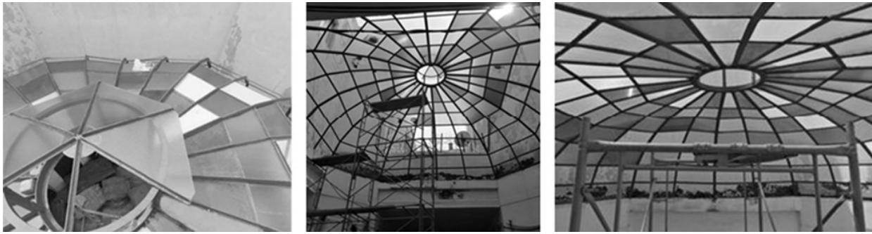
Figure 6. Left two Photos - the exterior and interior sides of Galleria Marriotti's dome during the process of adding colored plastic sheets. Source: OCTAB Facebook page (Accessed June 2020). Right-a photo of the interior side of the dome, uploaded by Hadia Gana to a Facebook post made by the author on June 13, 2020.
