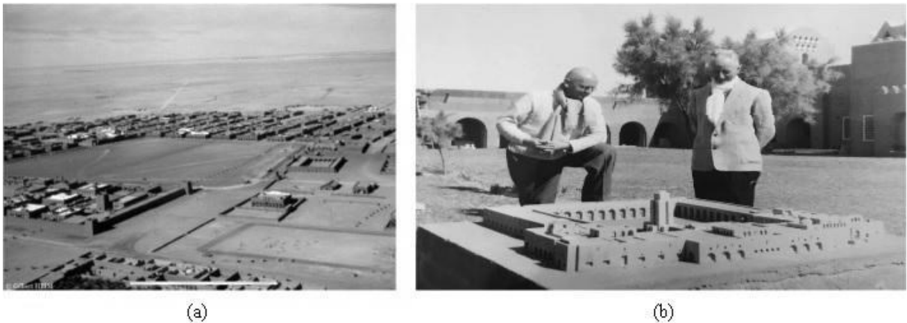
Figure 2: (a) Adrar Medina in colonial period, (b) Architect Michel Luyckx and architectural model of the historical hospital of Adrar
