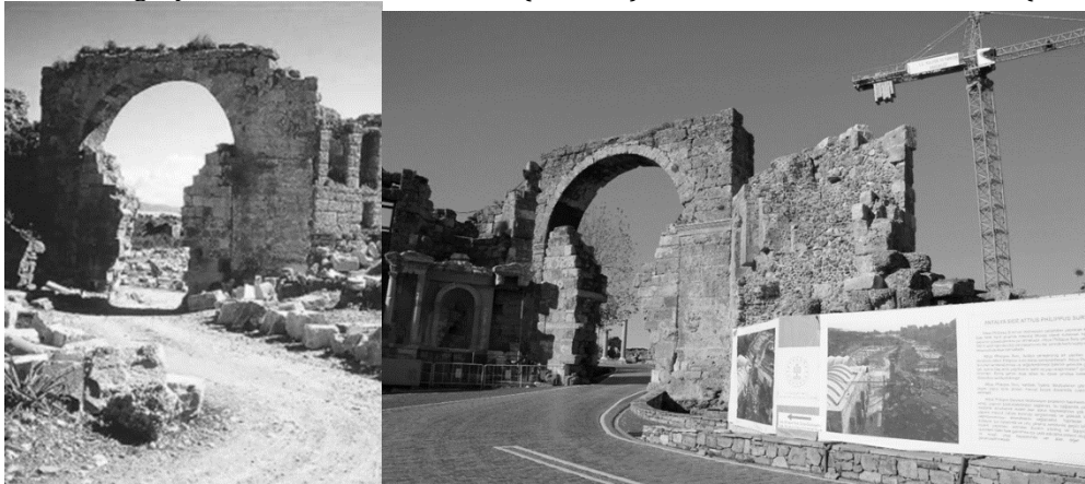
Figure 36 b. Pre-functionalization Tak (ÇŞİB)
