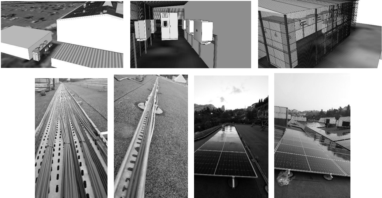
Figure 2. CarrefourSA İstinye SPP Project Execution Stages (From the Authors' Archive)
